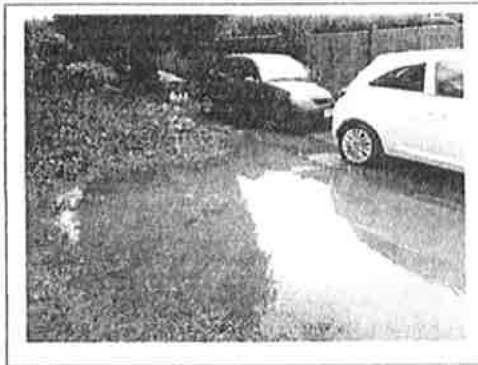
Stream overflows bank when pipe under drive becomes surcharged.
